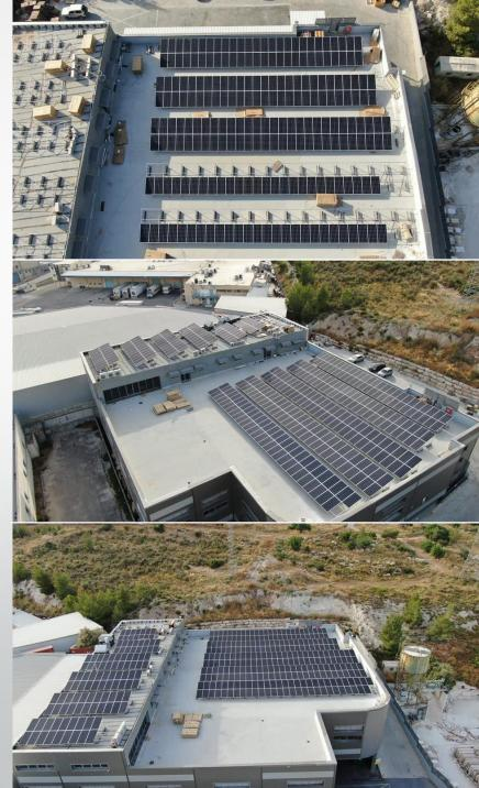
42KW system in Rosh-pina grid- connected with Solaredge — installed by an in-house team
